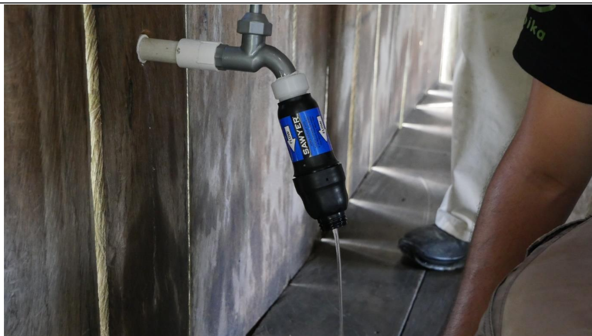
Sawyer micro-membrane filters installed in each household of San Juan de Los Parentes.
