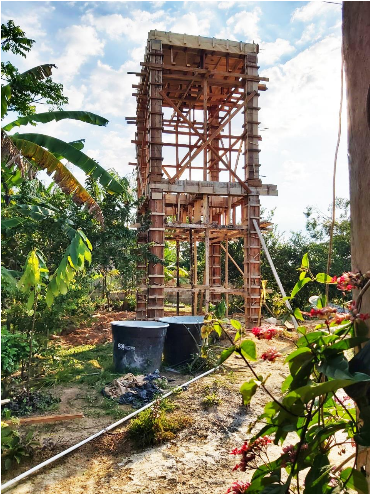
Example of some steps of the construction of the concrete tower.
