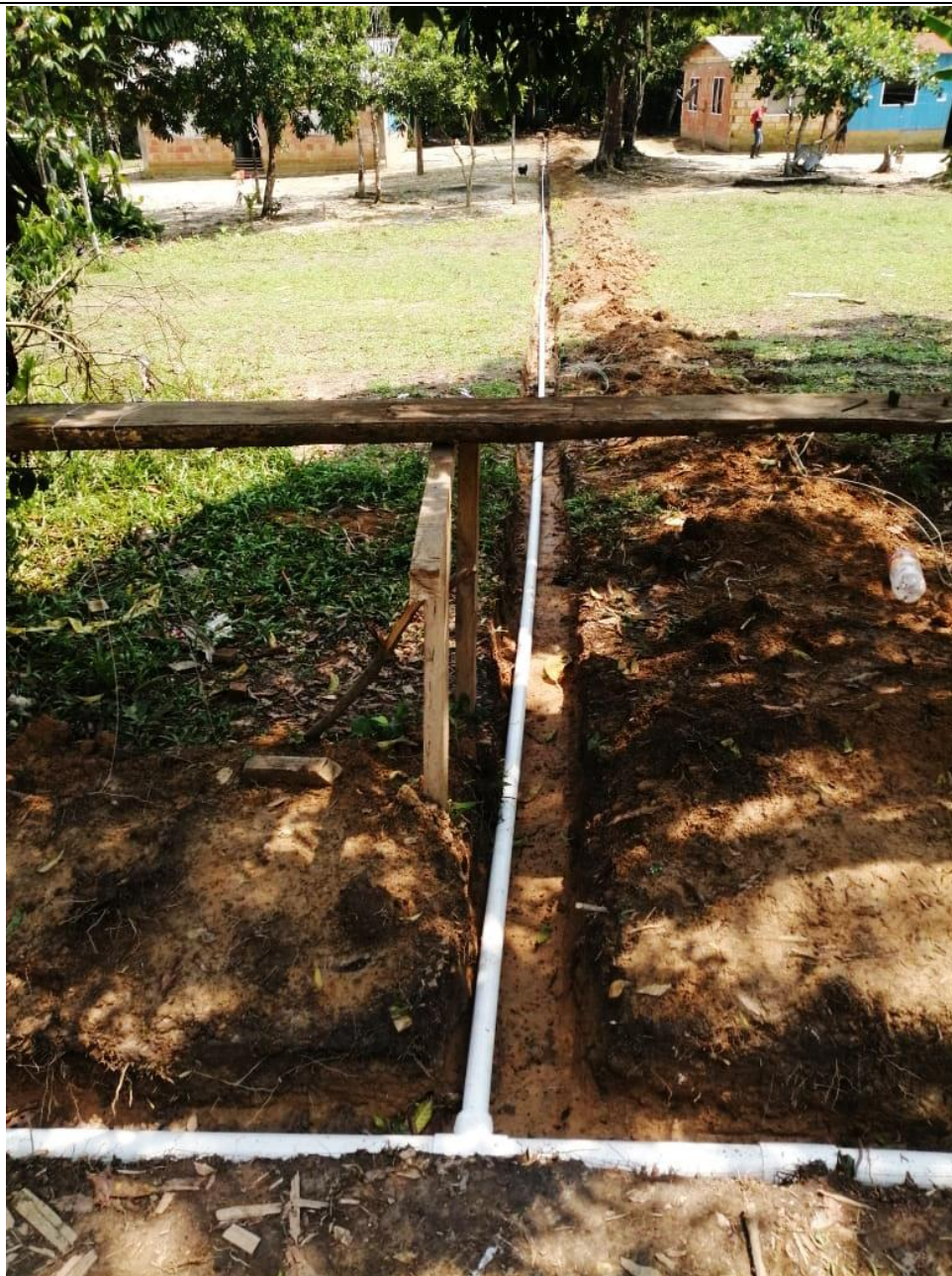
Example of the distribution network of pipelines reaching individual households.
